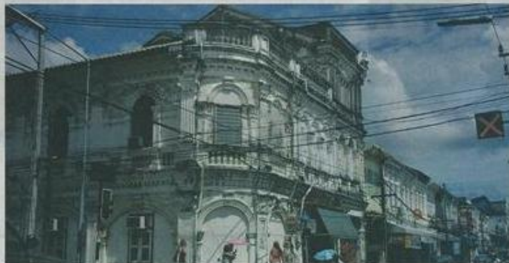
EFFORTS ARE under way to gentrify this part of Phuket town and to take down the unsightly aerial wires in the hope of drawing tourists from the beaches on the resort island to visit the urban area.
